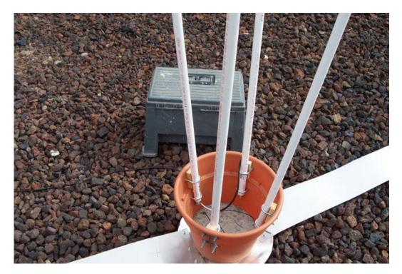
Concrete was poured into the bottom of the pot after four wires were connected to the through bolts to the bottom plate. These were covered with RTV before the concrete was poured. "U" bolts were used to connect the individual whips to the side of the plastic pot. The addition of the antenna switching network will go in the center above the concrete. Be sure to make drain holes so it doesn't collect water.
