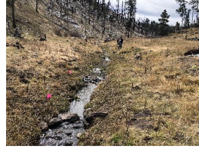
Work site with 1-rock dams and willow pole plantings
