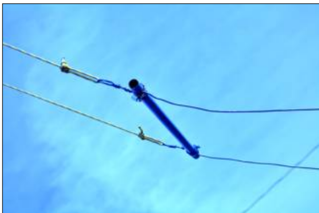
TFD end using 1/2" EMT tubing for conductive crossover connected to support ropes at mast ends.
