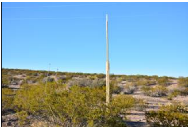
Building the wood support masts with 2"x4"x8½' and 8 ft. 2"x2s." Base support in concrete 2'6" ft. deep.
