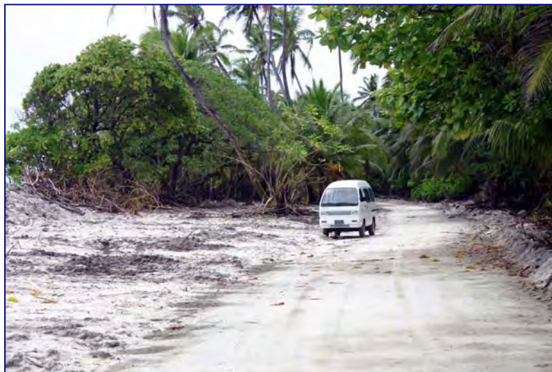
Figure 4.72 Graded area (Jan. 26, 2005).
