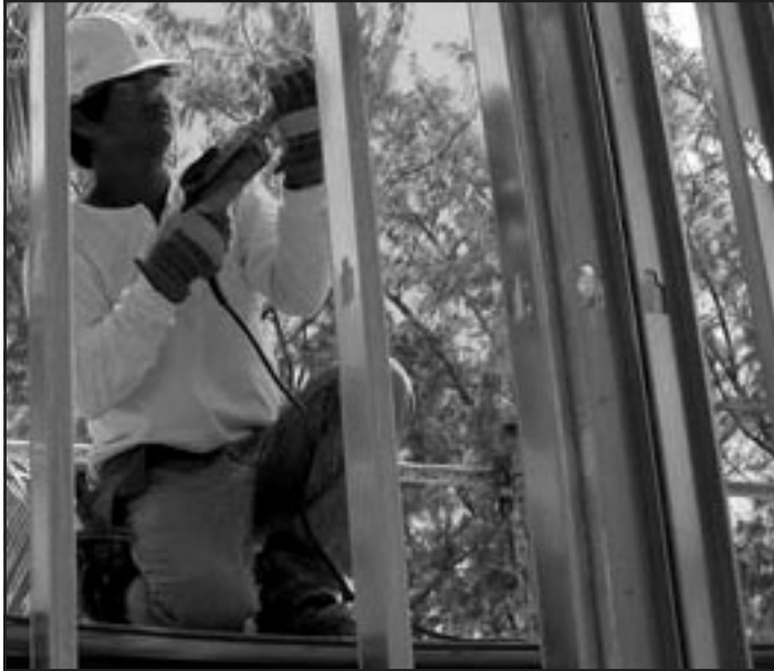
Leo Barbosa, of Manila, Philippines, installs a bit into an electric drill as he puts up wooden plates to strengthen the metal trussing for a new barracks-style housing unit being constructed at Splendidville Village.
