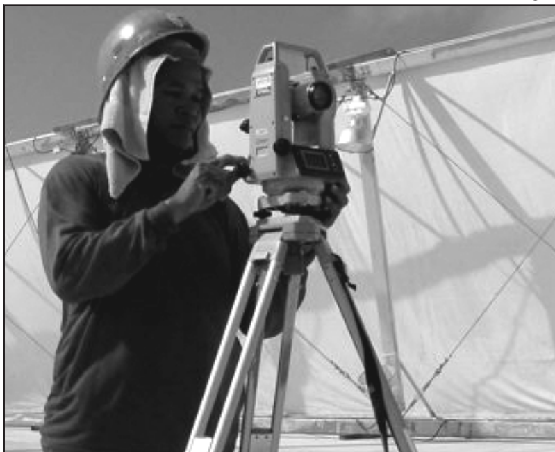
Cleto Arcangel, of Olongopo City, Philippines, prepares his equipment for aligning the surface slope for a new hangar bay. (Photo by JO2 Jeffrey Fretland, Naval Media Center)
