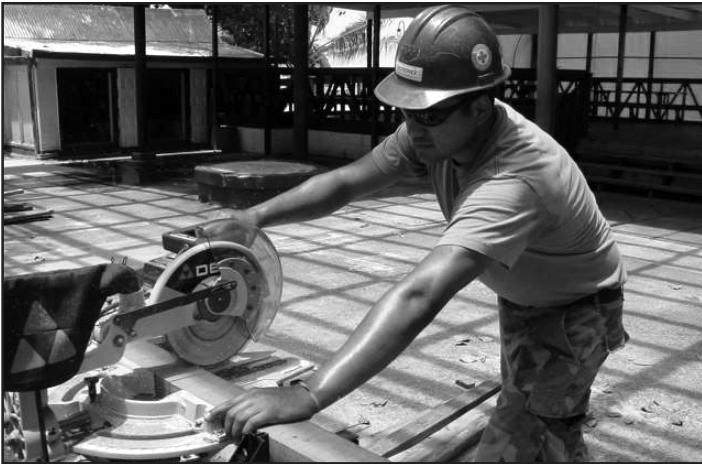
CE3(SCW) Joseph R. Quinonez, of Naval Construction Battalion 40, Port Hueneme, Calif., prepares to cut a two-by-four pine board for use as a bracing beam for the new Brit Club pavilion currently under construction.
