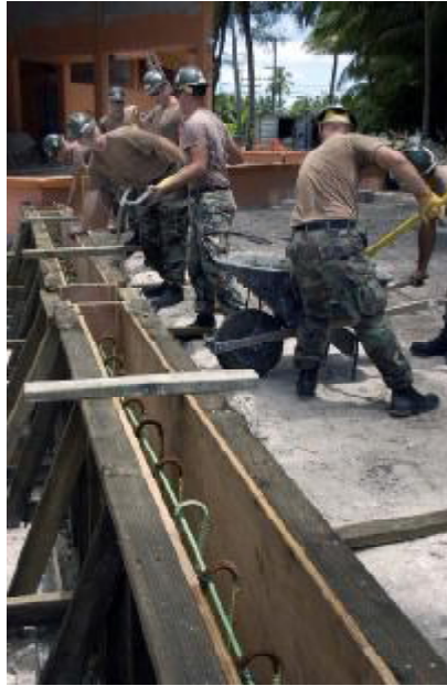
Forms had to be designed and assembled by the Seabees.
