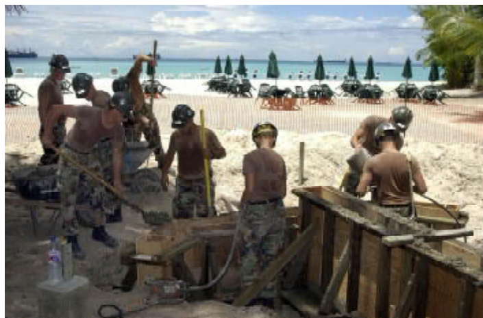
After weeks of preparations, the concrete is poured into the fabricated forms for deck supports.
