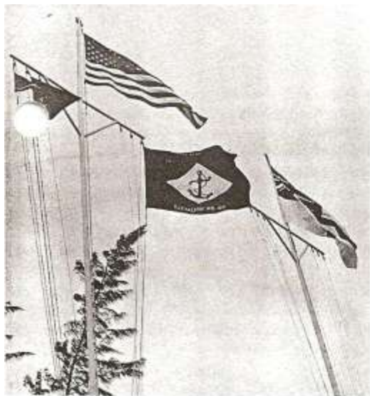
U. S. and British flags fly above the construction site of the joint communications station, with the builder's flag—NMCB-40—just below.
