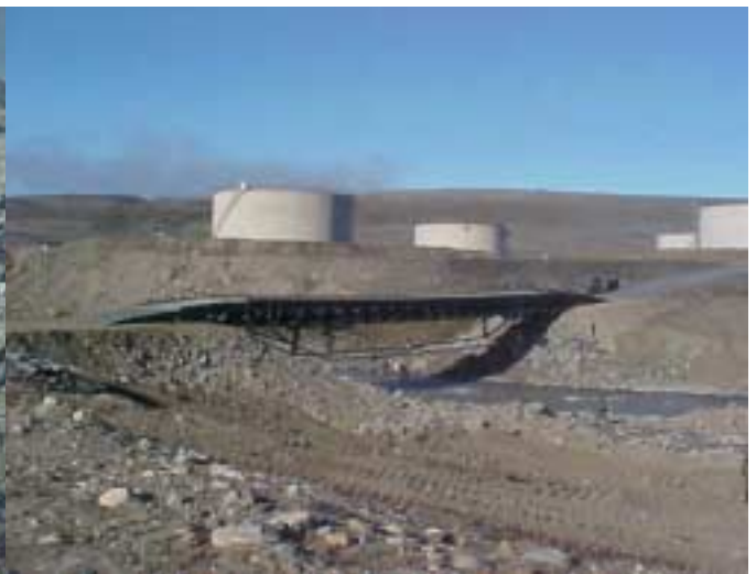
62nd Engineer Battalion, Ft. Hood, Texas finished product
