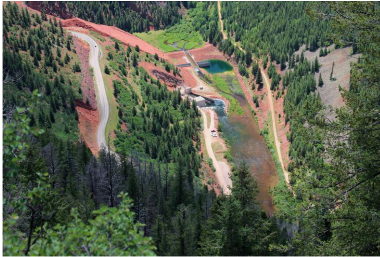
The Toilet Bowl and Upper Flats, Fryingspan River, Colorado
